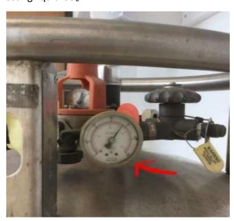
b. In the event that the pressure has dropped below 320 psig, gently open the Pressure Control valve to allow the pressure to increase. Close the Pressure Control valve once adequate pressure has been reached.
