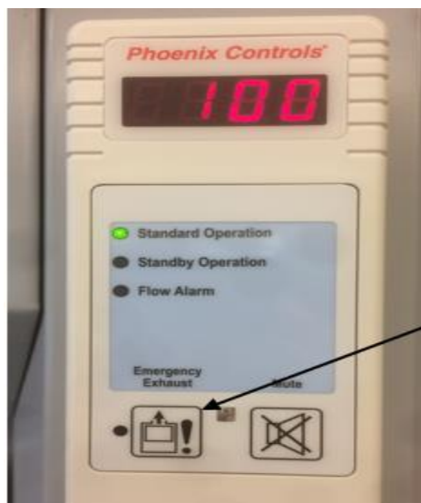
Figure 1: Black arrow shows the Emergency Exhaust button
